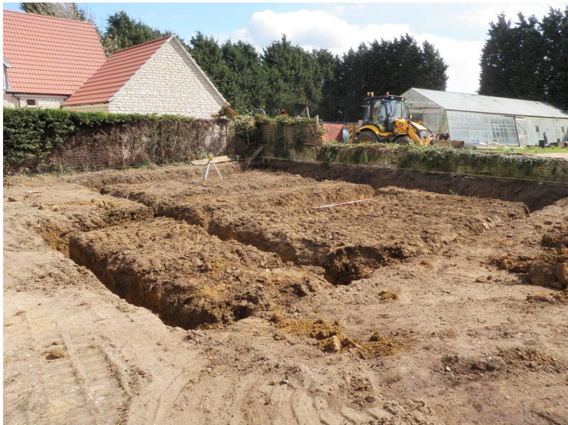
Plate 6 – Completed house footings, looking northeast
