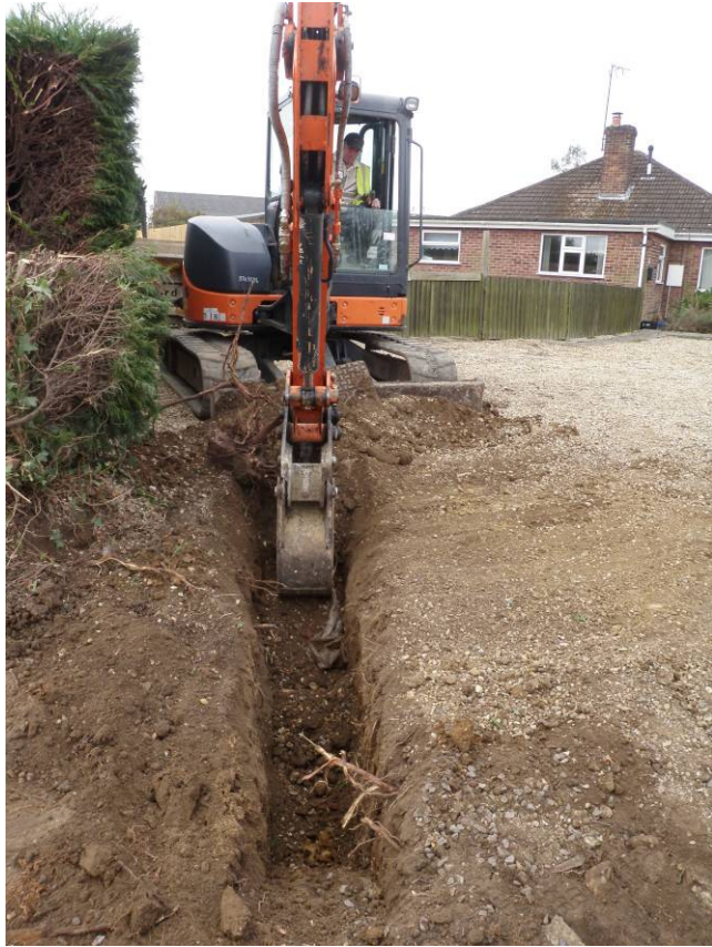
Plate 1 – Excavating service trench, looking south
