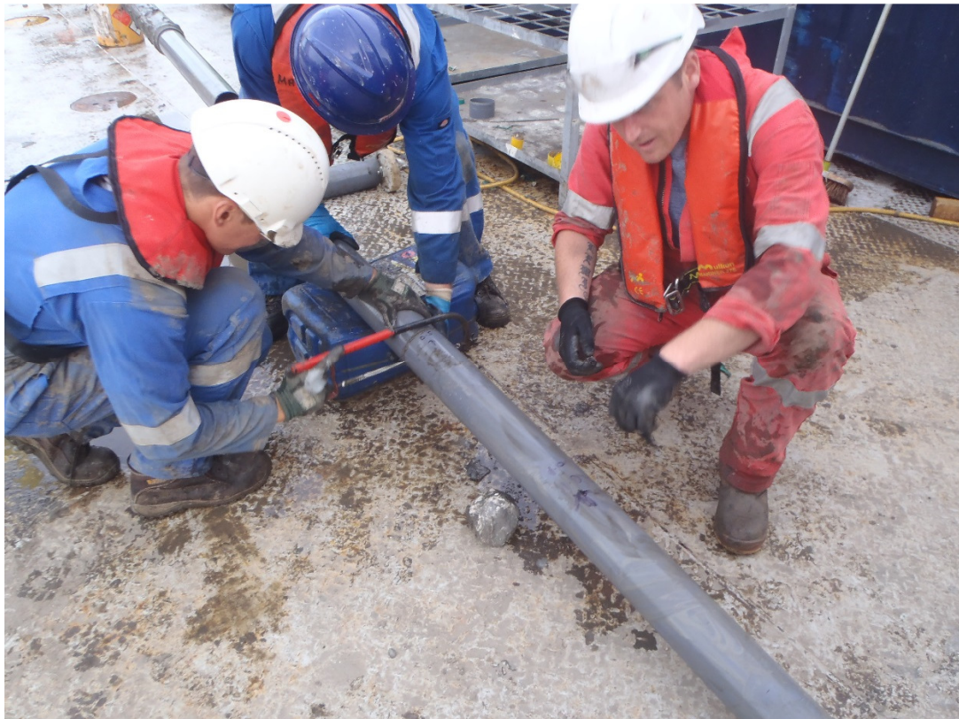
Plate 4. Cutting core from bore SC 1
