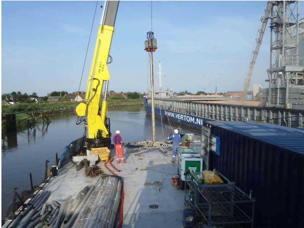
Plate 1. The general rig set-up seen from the bridge
