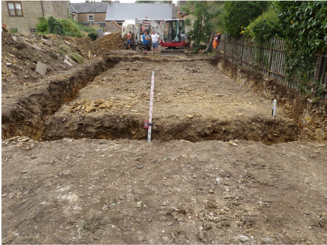
Plate 5, Post-excavation, looking west
