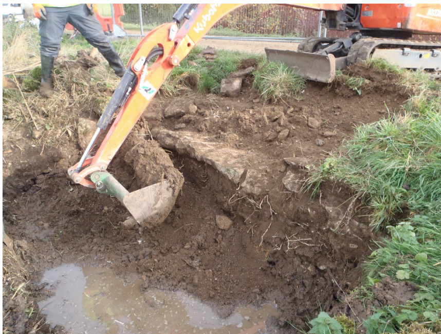
Plate 4 – Excavation of the recess behind Arch 12
