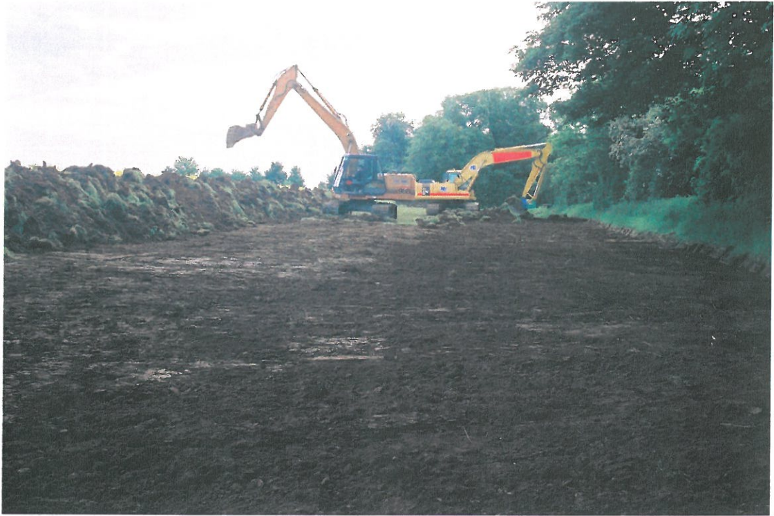
Plate 1 General view showing methodology for stripping of topsoil from easement
