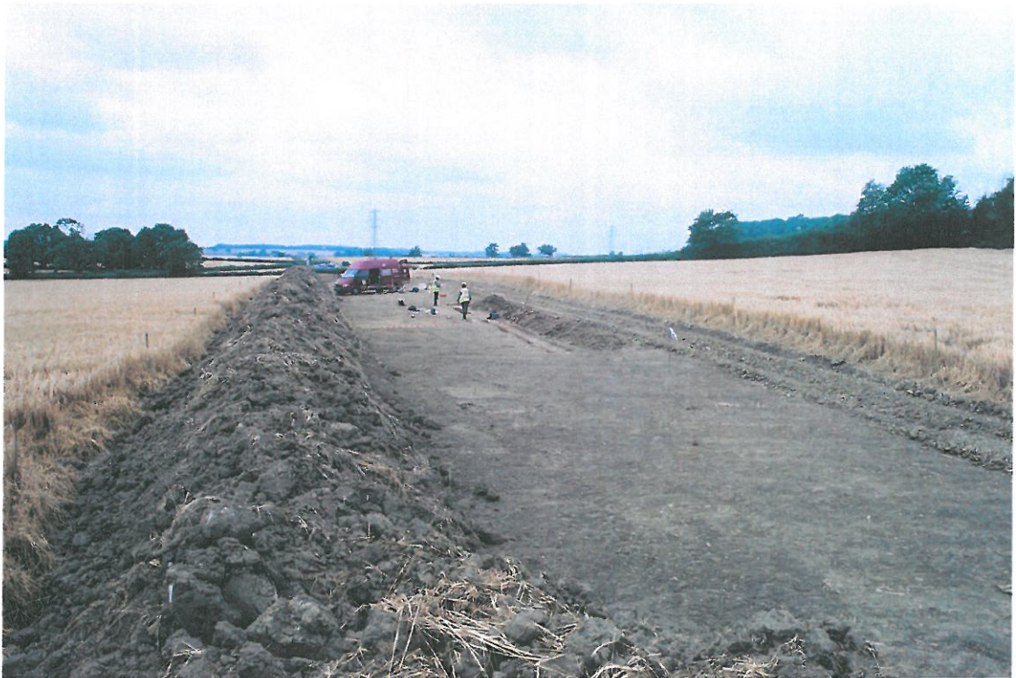
Plate 20 Area 3, general working view, looking west
