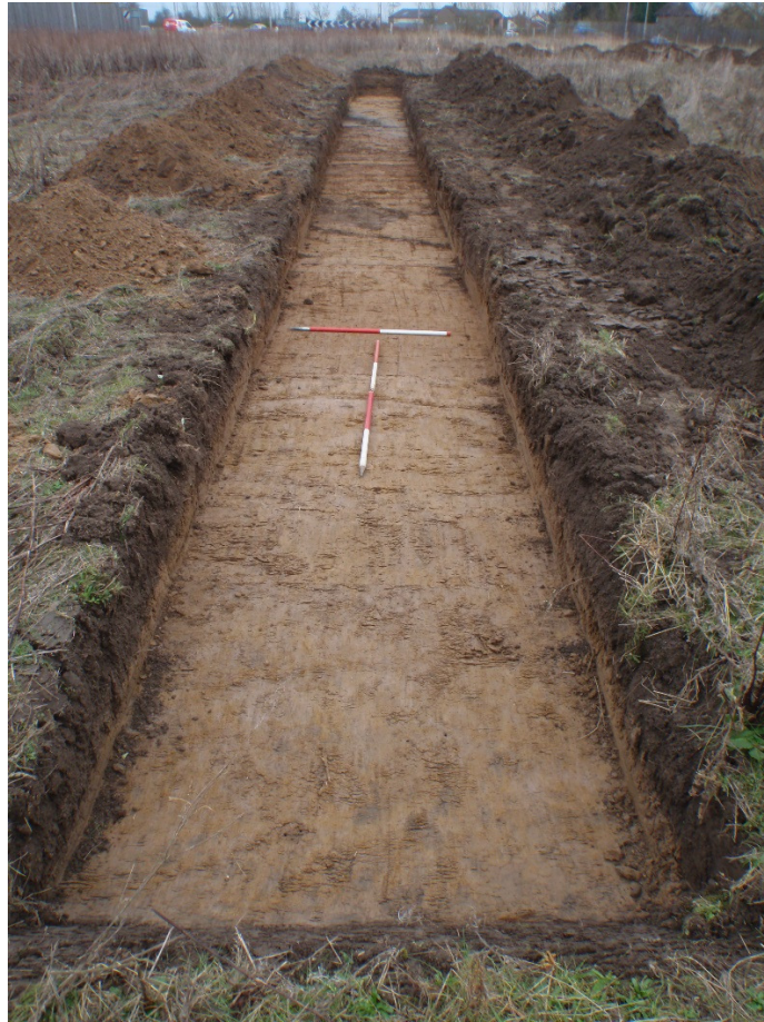
Plate 5 – Trench 2 after machine excavation, looking northeast
