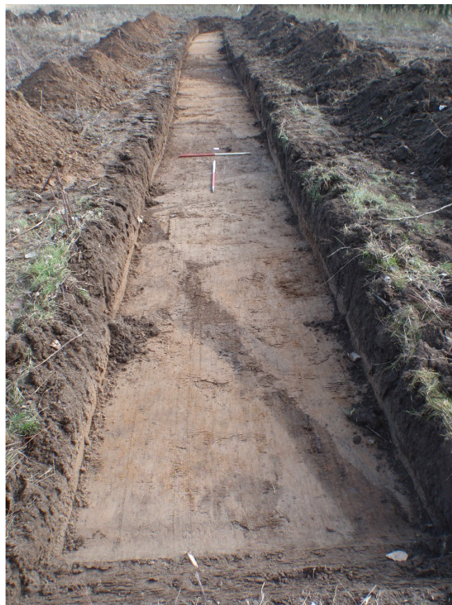
Plate 2 – Trench 1 after machine excavation, looking southeast
