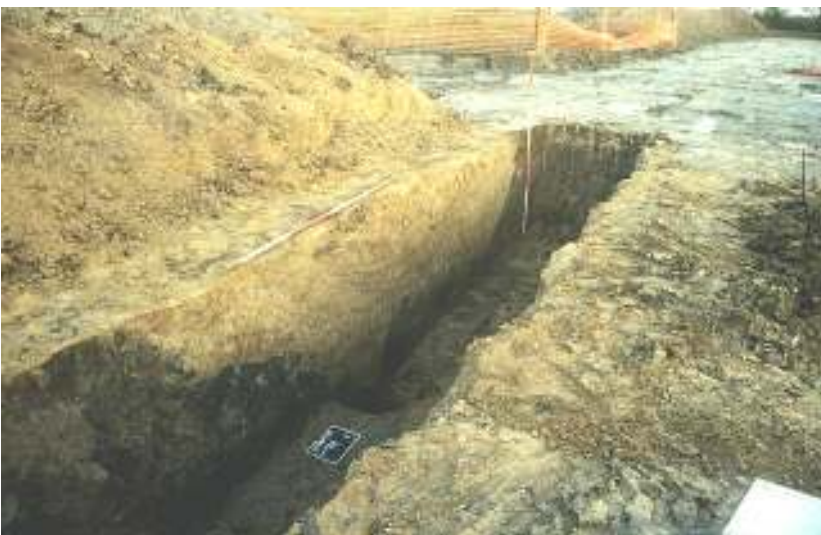
Plate 15 - RWP299: Section 44 showing ditch/creek (393), looking northeast
