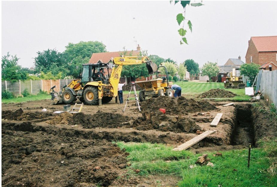
Plate 1 – General view of the development area, looking north
