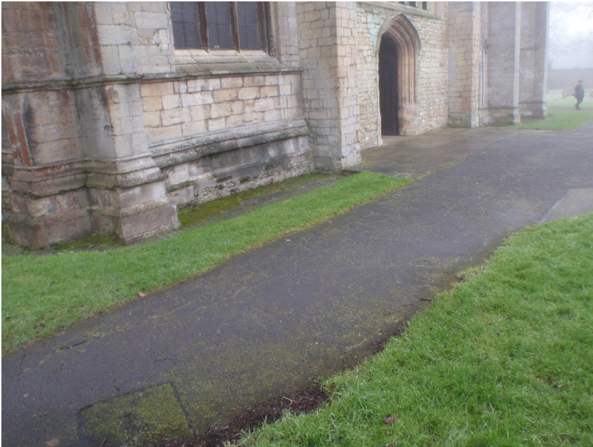
Plate 1 – General view of the west end of the church, prior to excavation, looking southeast
