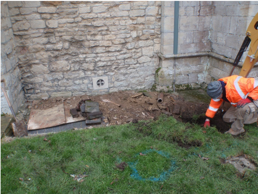
Plate 2 – General view of the works in progress, looking east
