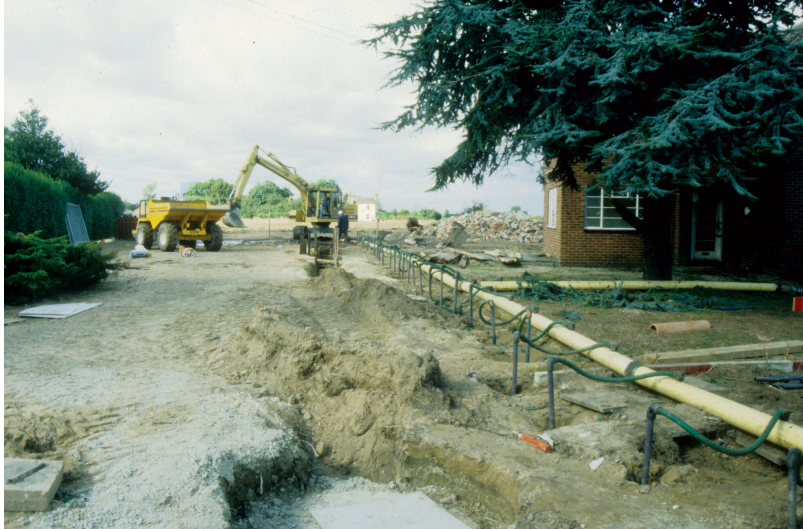
Plate 1 – General view looking west across the site
