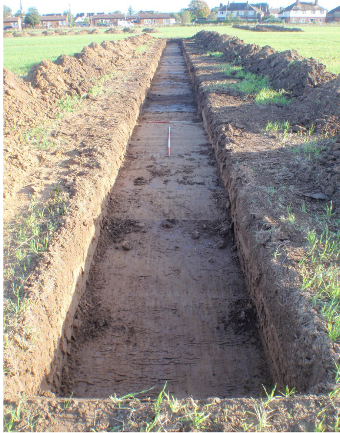
Plate 3 – Trench 2 after excavation, looking north
