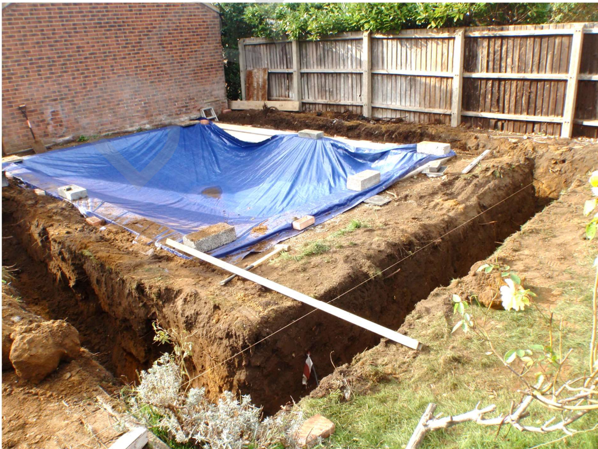
Plate 5. General view of the footings, looking northwest
