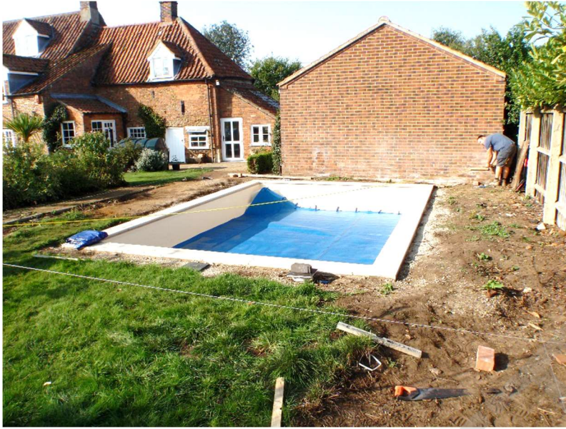
Plate 1. The site, prior to the excavation of the footings, looking southwest
