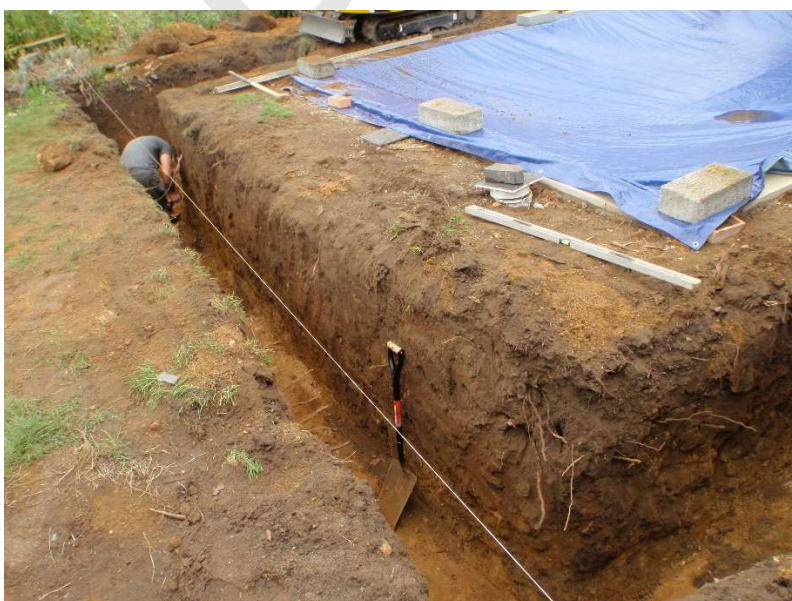
Plate 3. Excavating the footings, looking south
