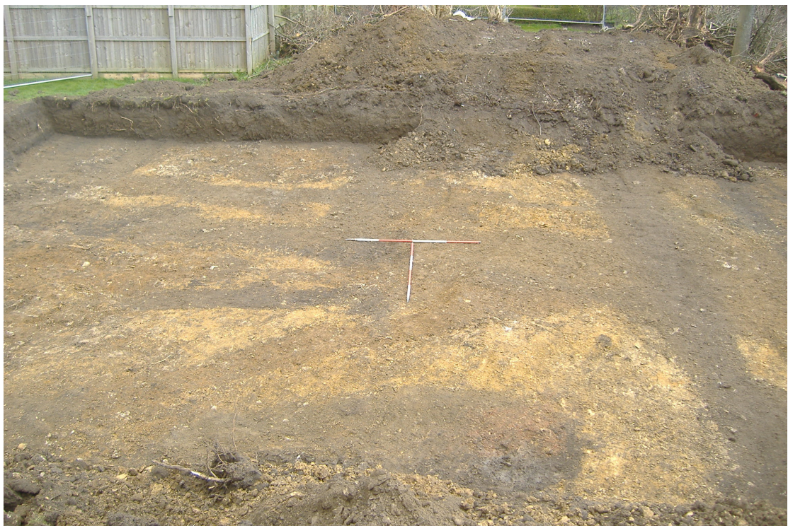
Plate 2 – The eastern half of the site prior to excavation, looking east
