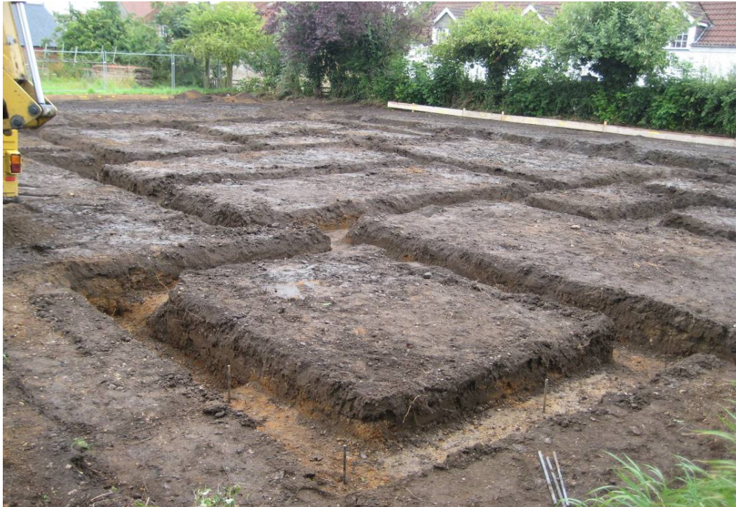
Fully excavated footings looking east
