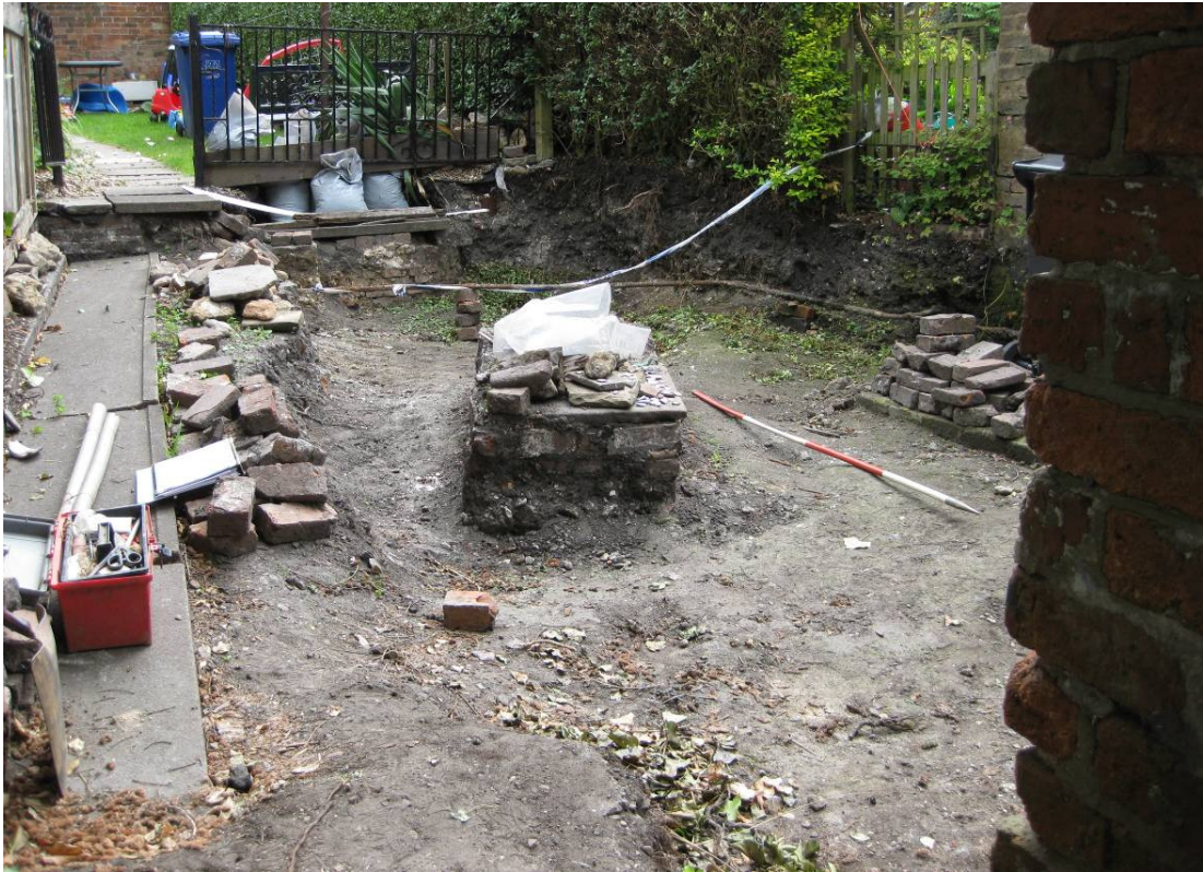
Plate 1 – General view of area of ground reduction looking north
