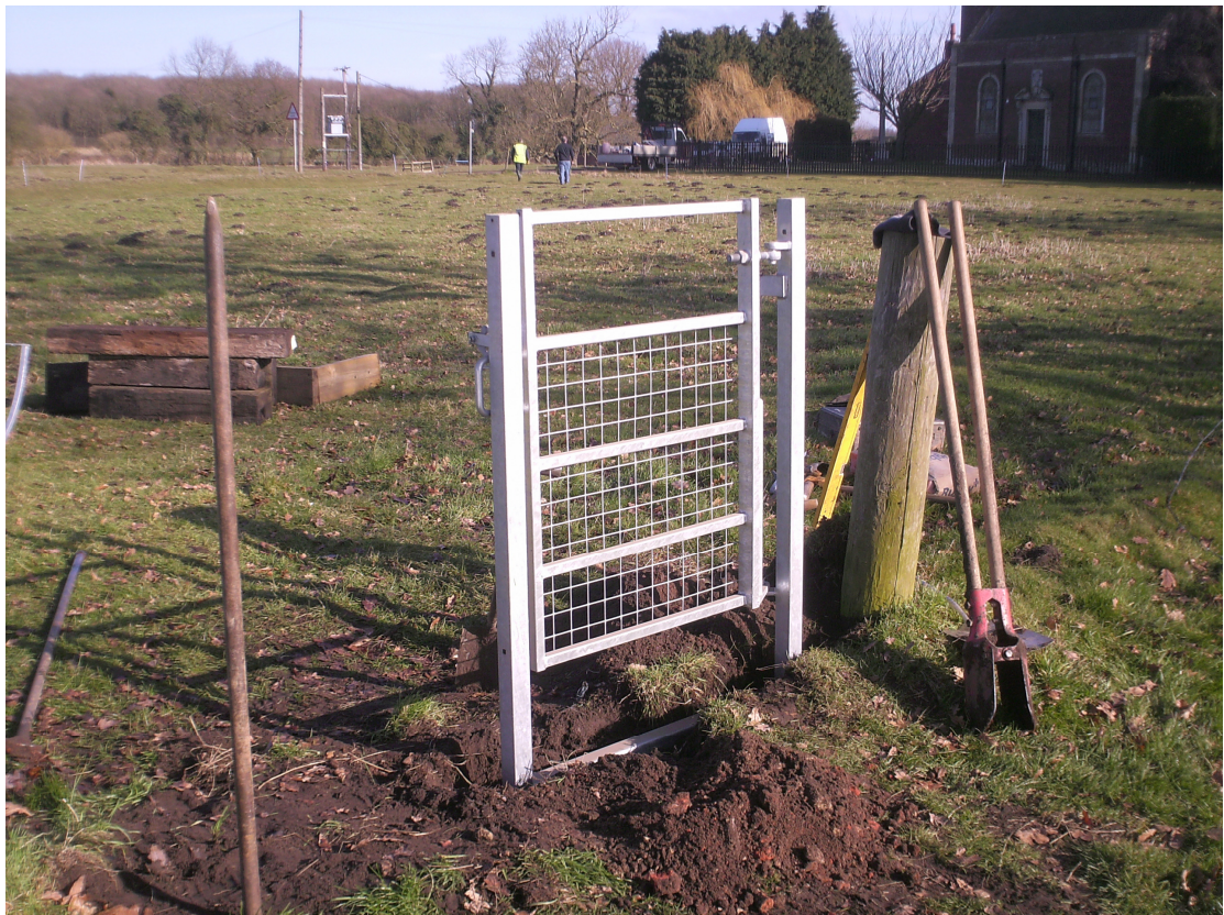
Plate 2 – Installation of the kissing gate, looking northeast
