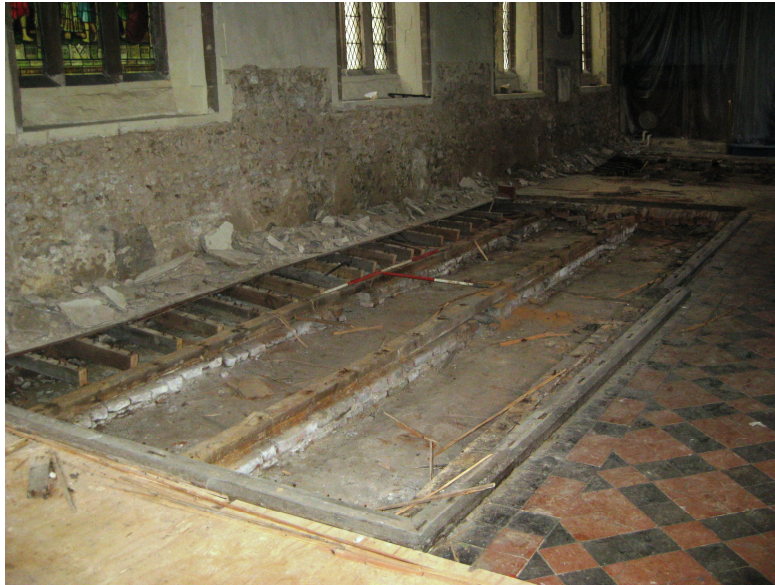
Plate 1 – General view of the area of works, looking northeast
