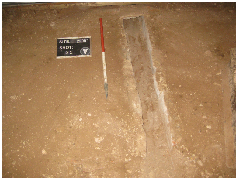
Plate 4 – View of the air duct (012), looking south
