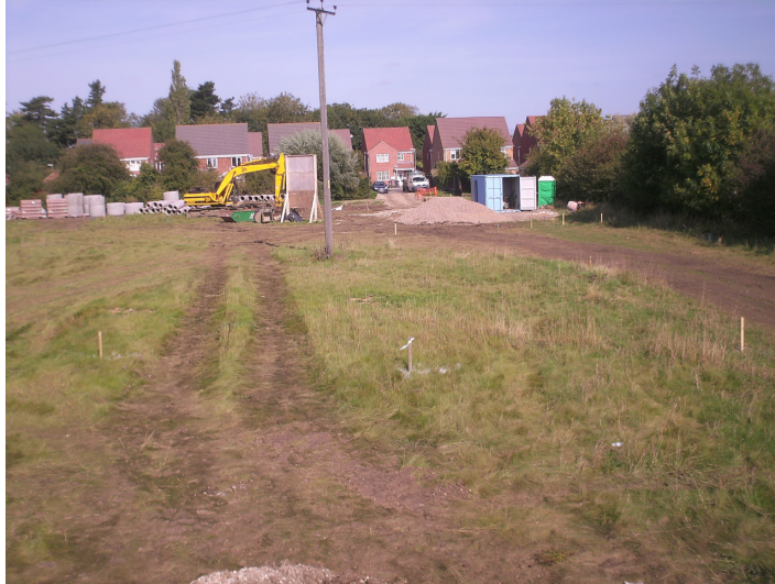
Plate 1 – General view looking north over the development site
