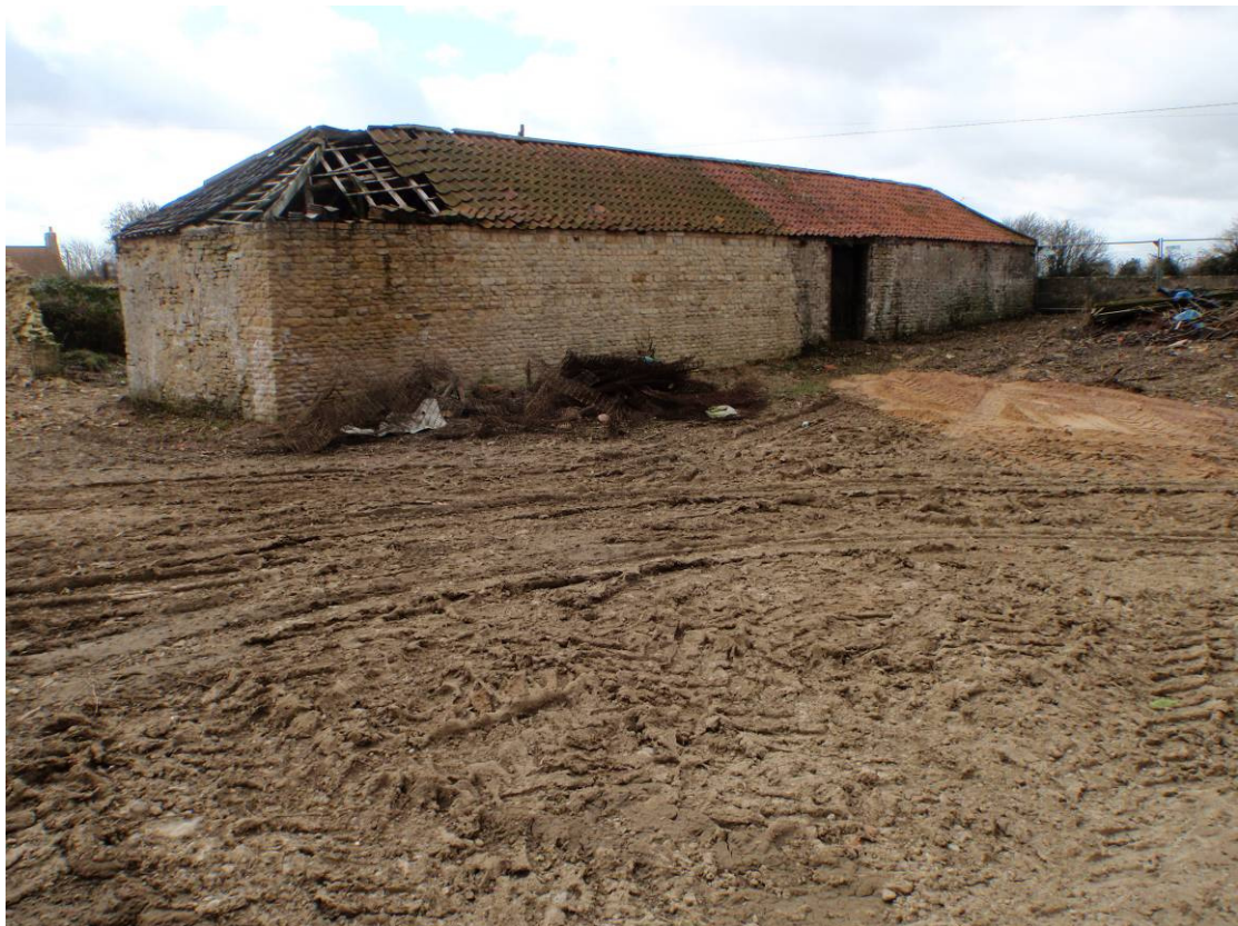
Plate 22 – Building 3 - North side of cowhouse, looking southwest
