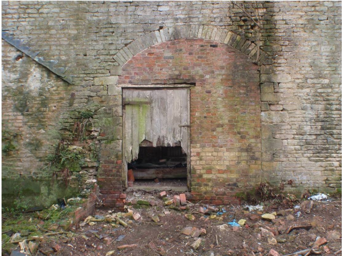
Plate 3 – Building 1 - East side of barn, main door, looking east
