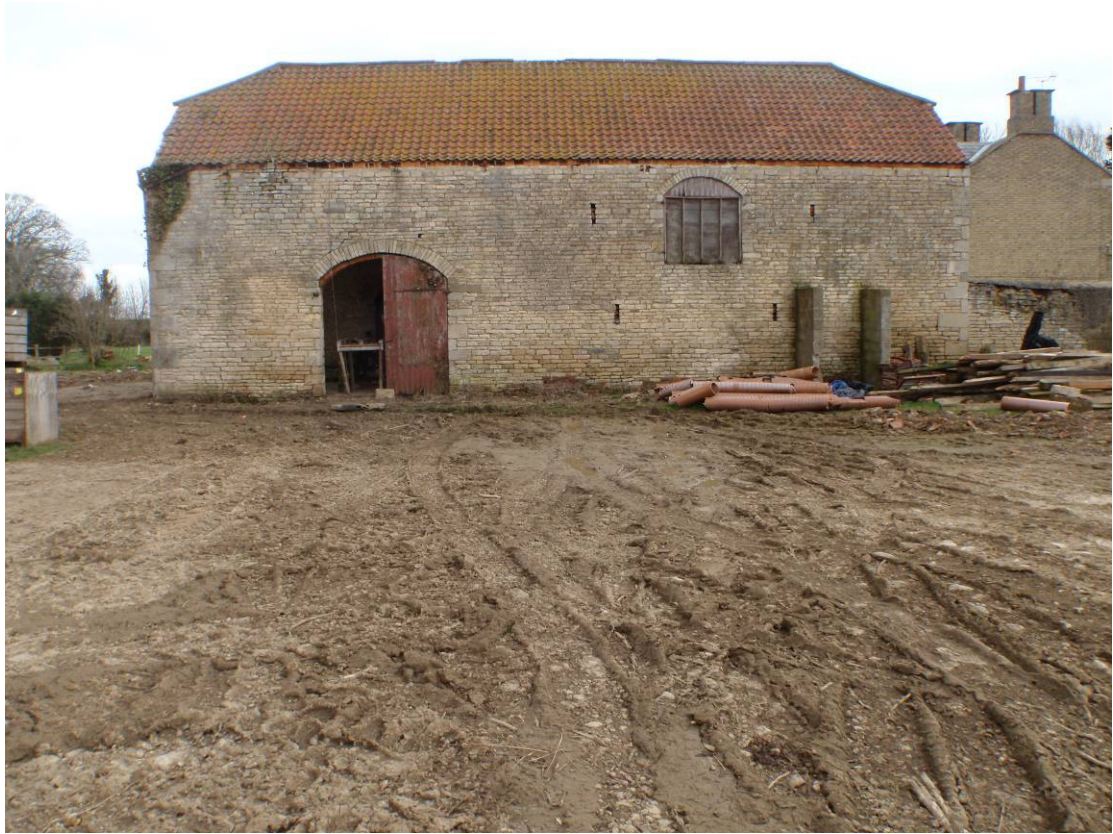
Plate 5 – Building 1 - West side of barn, looking east
