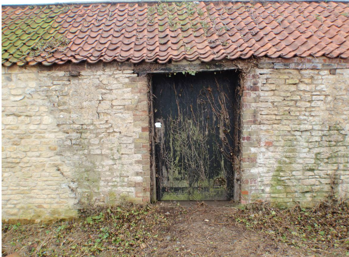
Plate 24 – Building 3 - North side of cowhouse, door, looking south
