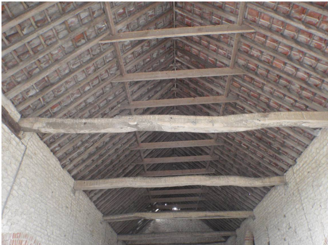
Plate 8 – Building 1 - Interior of barn, roof, looking south
