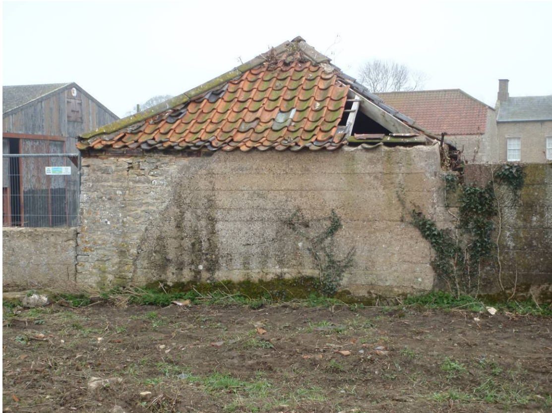
Plate 21 – Building 3 - West side of cowhouse, looking east
