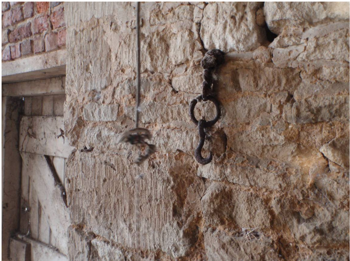
Plate 12 – Building 1 - Interior of barn, iron fitting in east wall, looking northeast
