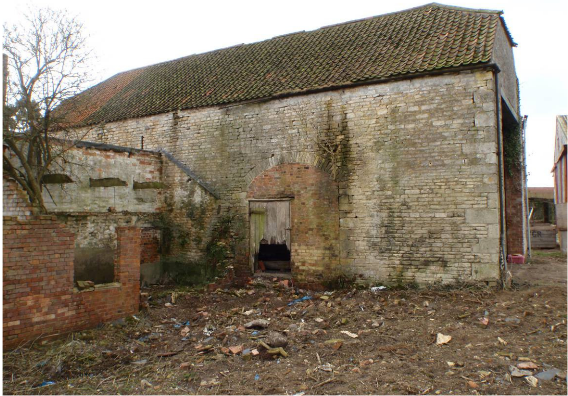
Plate 7 - Building 1 - East side of barn, looking west-southwest
