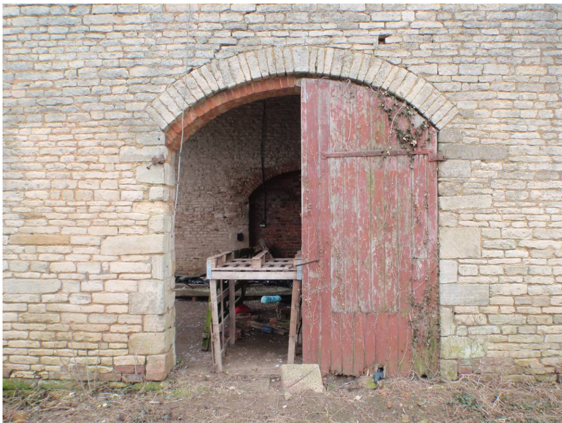
Plate 2 – Building 1 - West side of barn, main door, looking east
