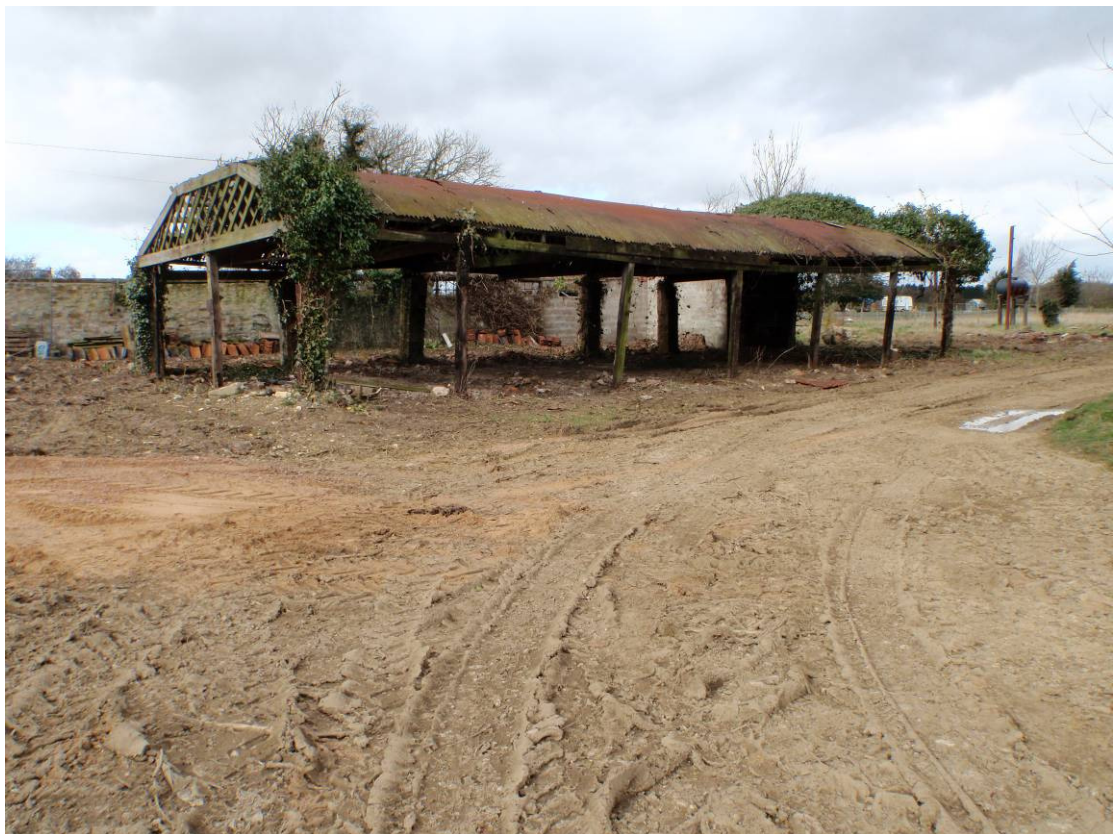
Plate 37- Other buildings - Open structure north of the cowhouse, looking northwest
