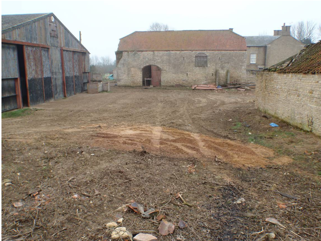
Plate 1 – Building 1 - West side of barn, cowhouse and modern shed, looking east
