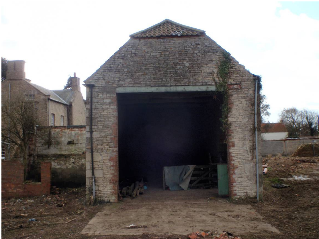
Plate 6 - Building 1 - North side of barn, looking south
