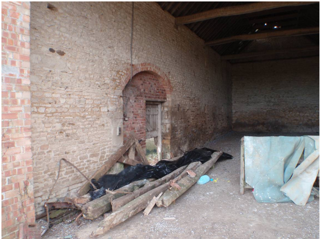
Plate 14 – Building 1 - Interior of barn, east wall, looking southeast
