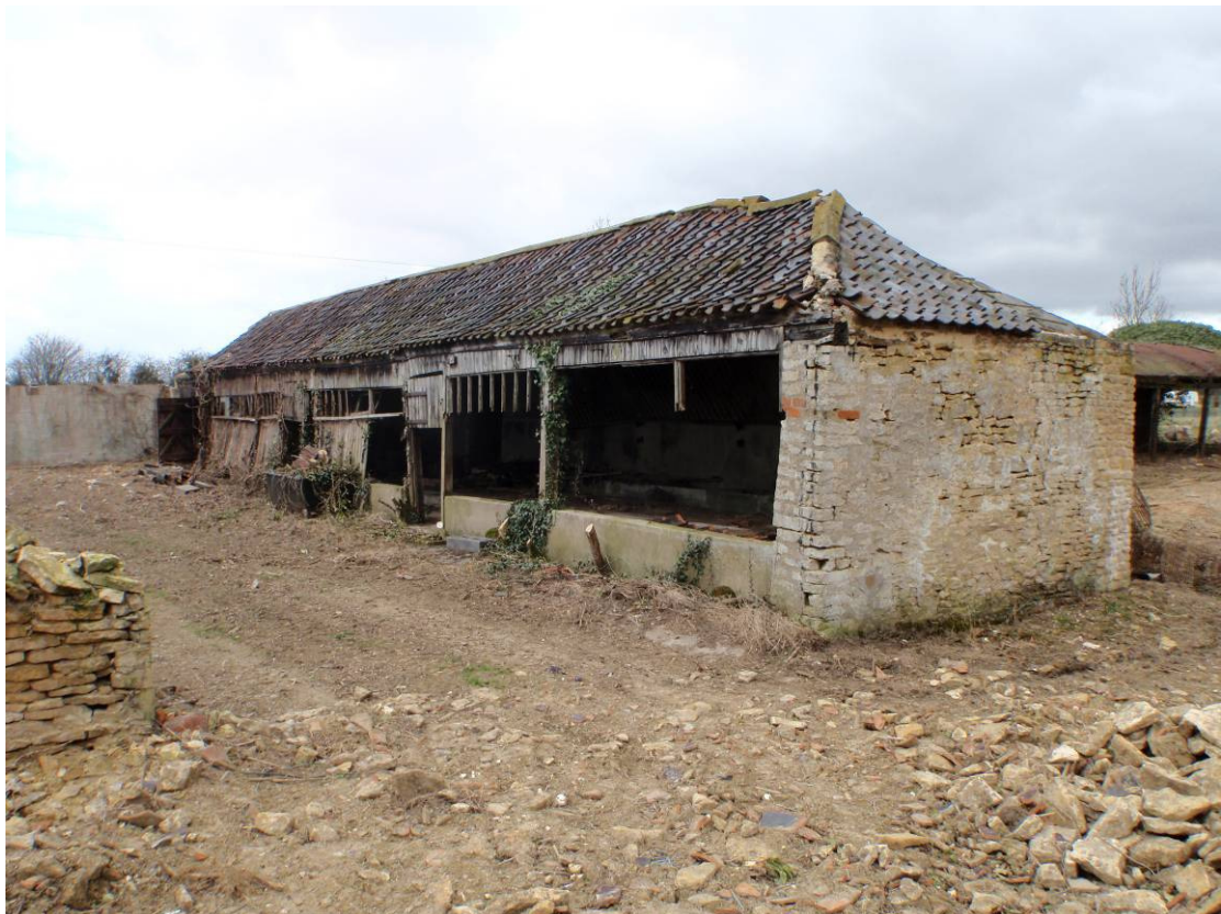
Plate 26 – Building 3 - South side of cowhouse, looking northwest
