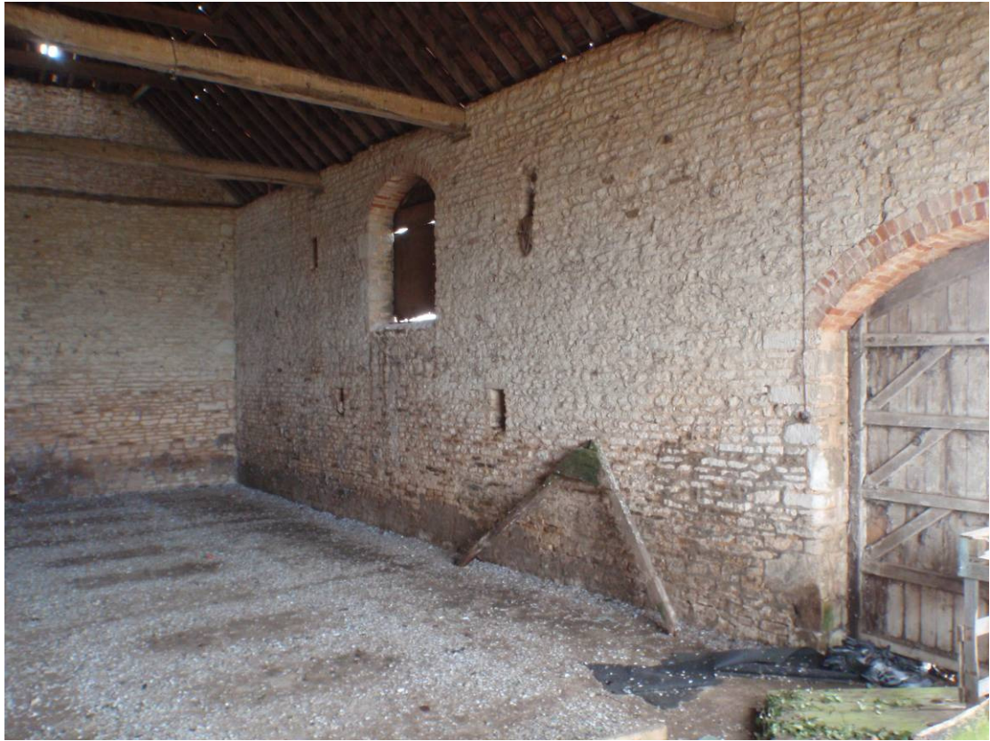
Plate 13 – Building 1 - Interior of barn, west wall, looking southwest
