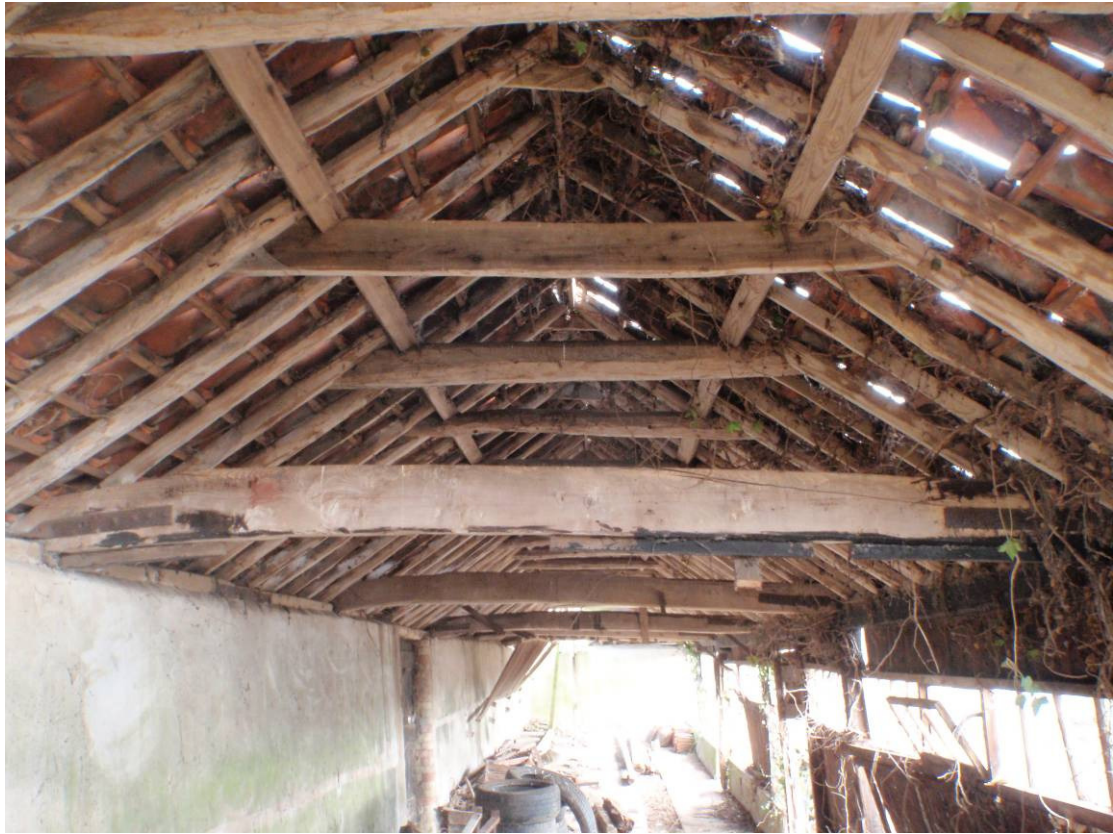
Plate 25 – Building 3 - Interior of cowhouse, roof, looking east
