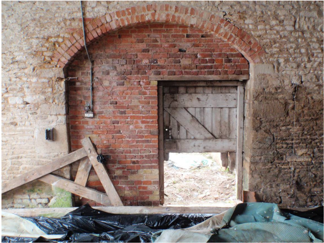
Plate 9 – Building 1 - Interior of barn, east door, looking east
