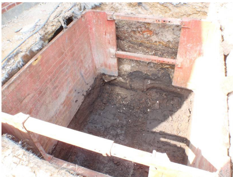
Plate 15. Rainwater tank pit dug to full depth showing deposit 040
