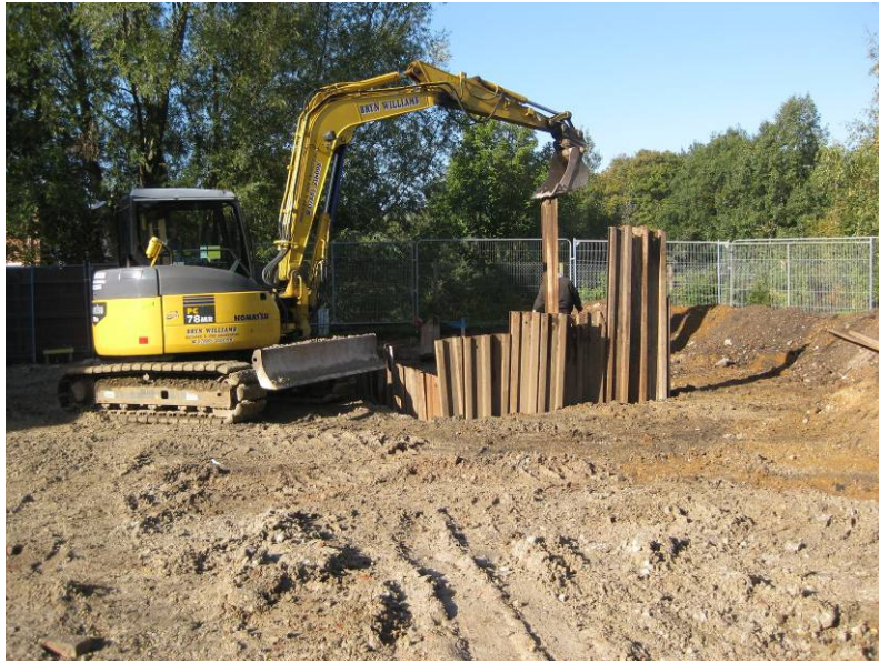
Plate 4. Pushing in the Trench 1 shoring, looking northwest
