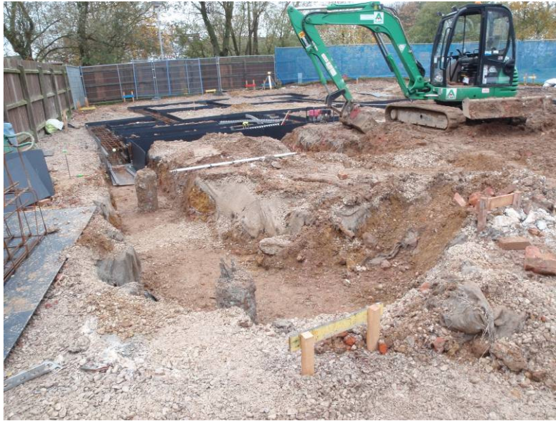
Plate 10. View of footings on watching brief looking west
