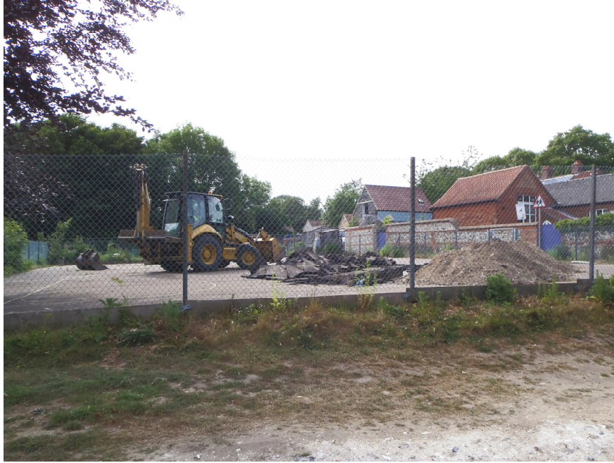
Plate 1 – General view across the development area, looking west
