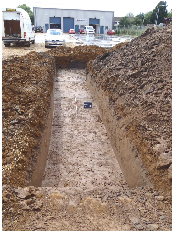
Plate 3 – The eastern part of the trench after cleaning, looking south
