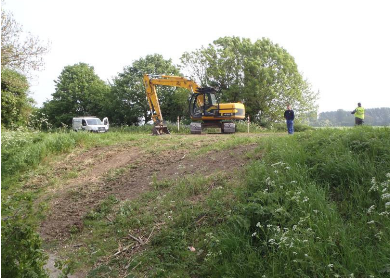
Plate 1 – General view of the area prior to excavation, looking northeast
