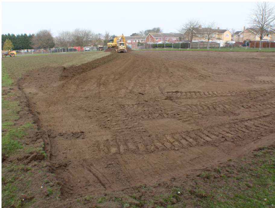
Plate 2 General view of site during topsoil strip, looking north
