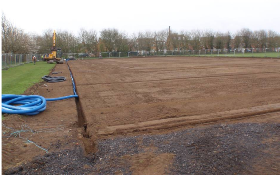
Plate 4 Perimeter drainage ditch, looking south
