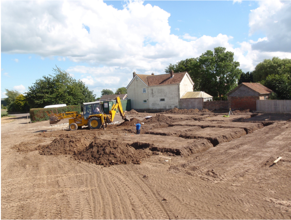
Plate 1: The foundation trenches
