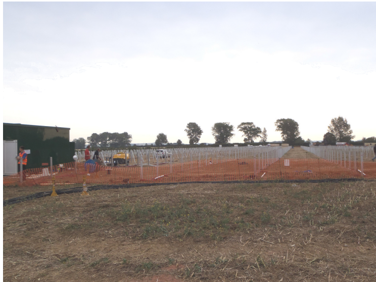
Plate 1 – General view across the site, looking northeast
