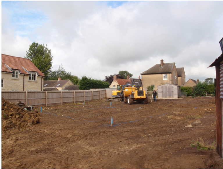
Plate 1 – General view of the development area, looking west
