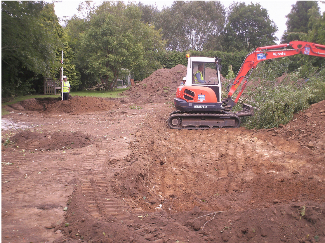
Plate 5: Stripping the remainder of the development area
