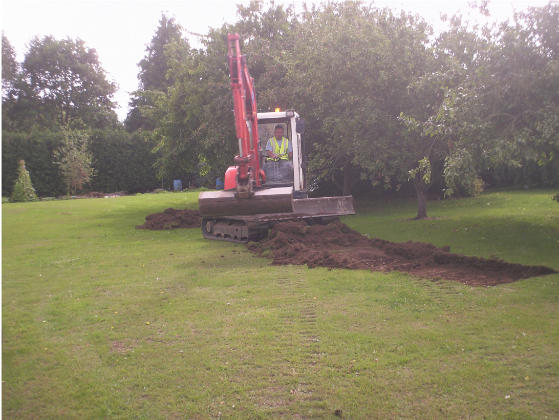
Plate 1: Location of Trench 1
