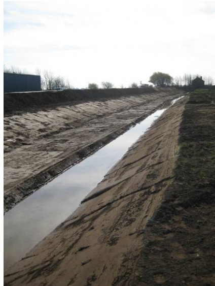
Plate 1 – General view of drainage ditch
