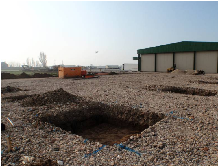
Plate 5 – General view of stanchions in area of new building
