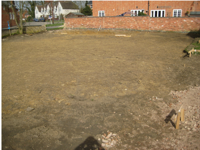
Plate 1 – General shot looking over Plot 1, looking northwest
