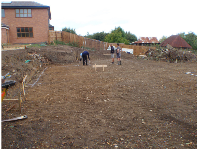
Plate 5 – View looking over the area of Plot 3, looking east
