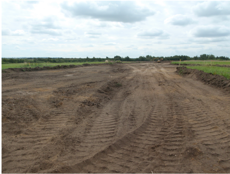
Plate 4 – View along the road strip area from Whisby Road, looking south
