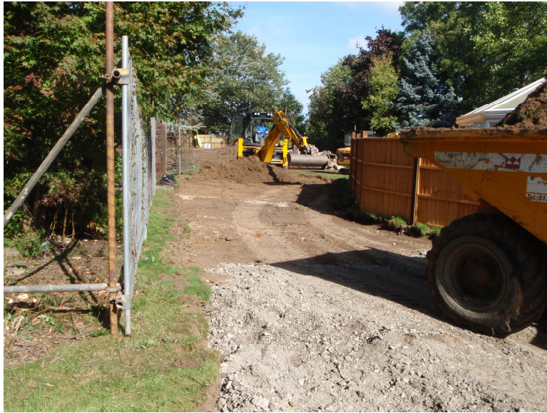
Plate 1. Road stripping in progress looking north
