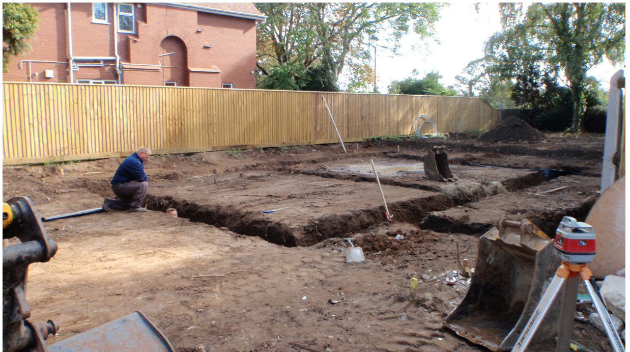
Plate 5. Plot 1 footings looking southeast
