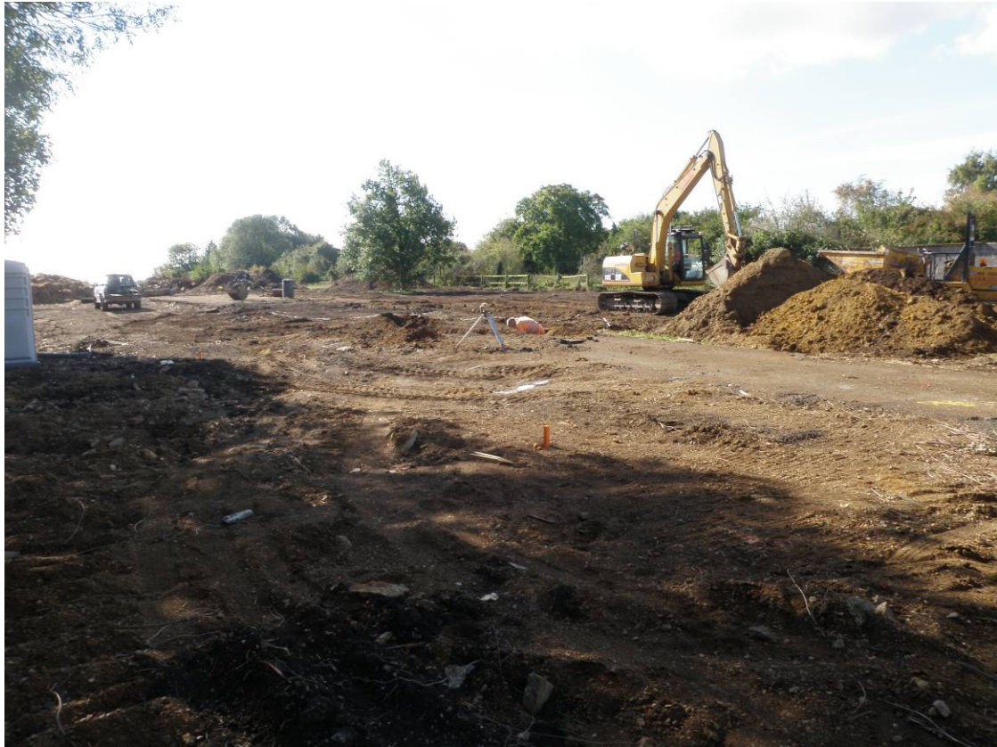
Plate 1. General view of site looking south
