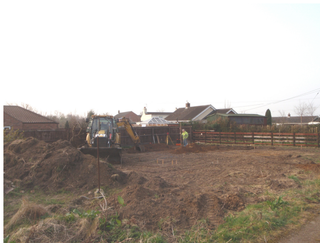
Plate 2 – The garage plot during excavation, looking south
