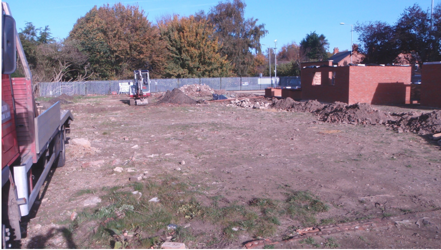
Plate 1 – General view of the development area, looking north
