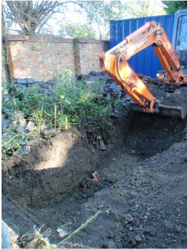
Plate 1 – Excavation of Trench 1 in progress
