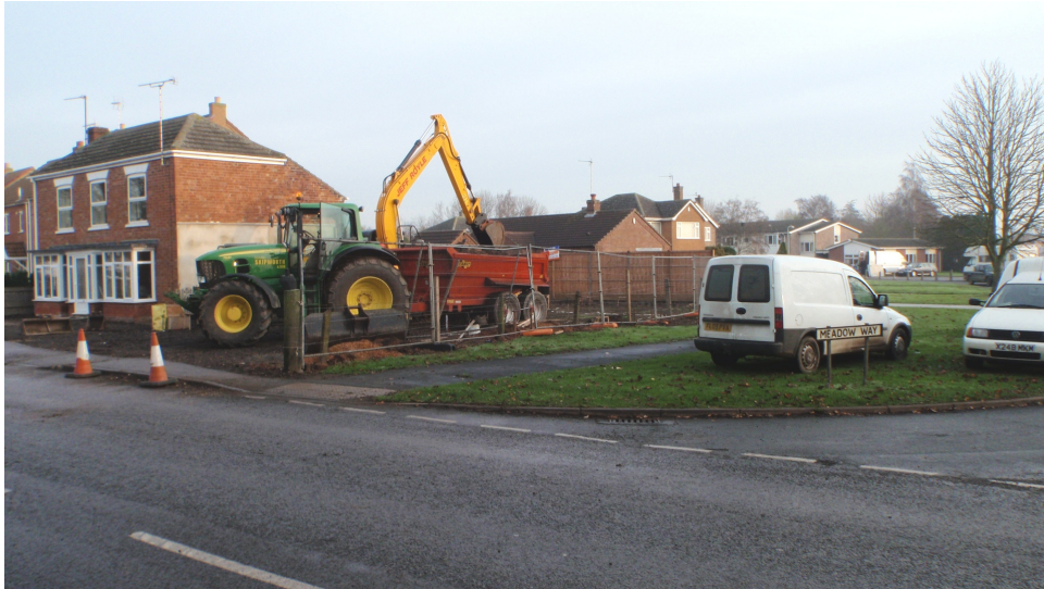
Plate 1 – General view of the development area, looking northeast
