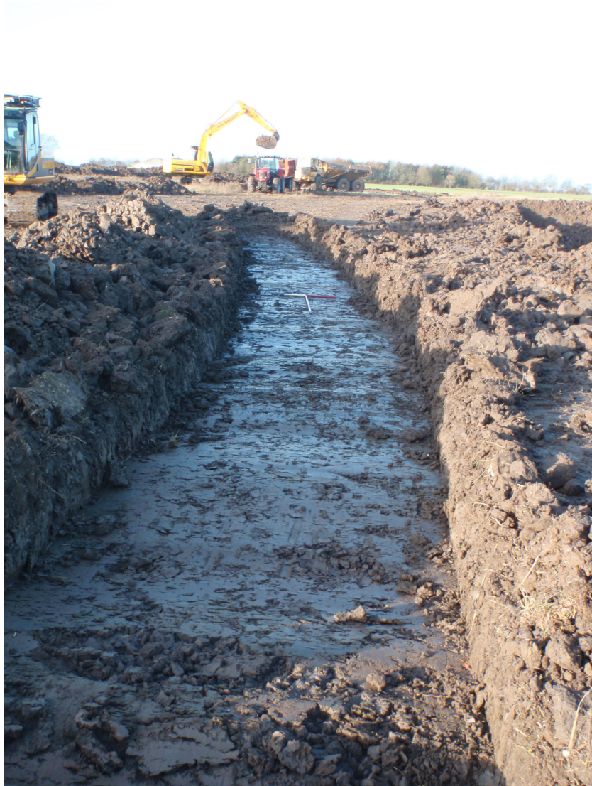
Plate 7: Trench 3 - general shot
