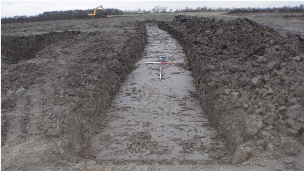
Plate 6: Trench 2 - general shot
