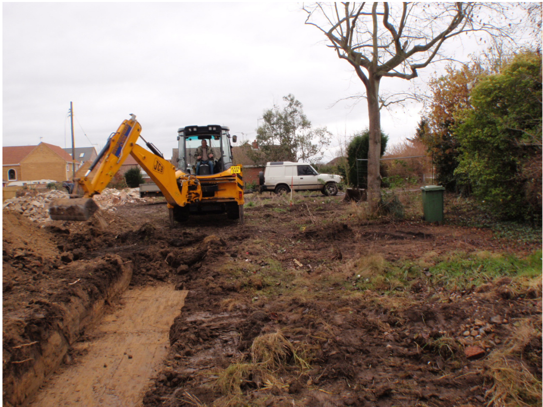
Plate 2. Machining Trench 2 looking east
