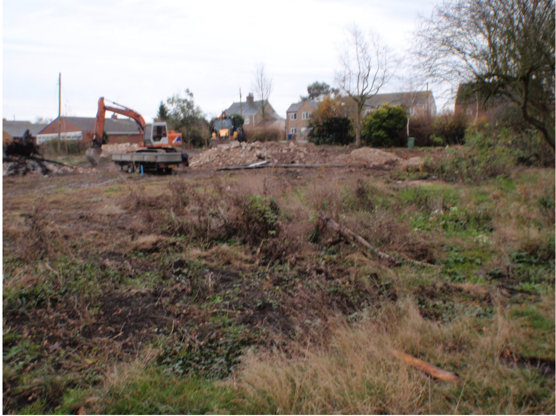
Plate 1. Pre-machining view of site looking southeast
