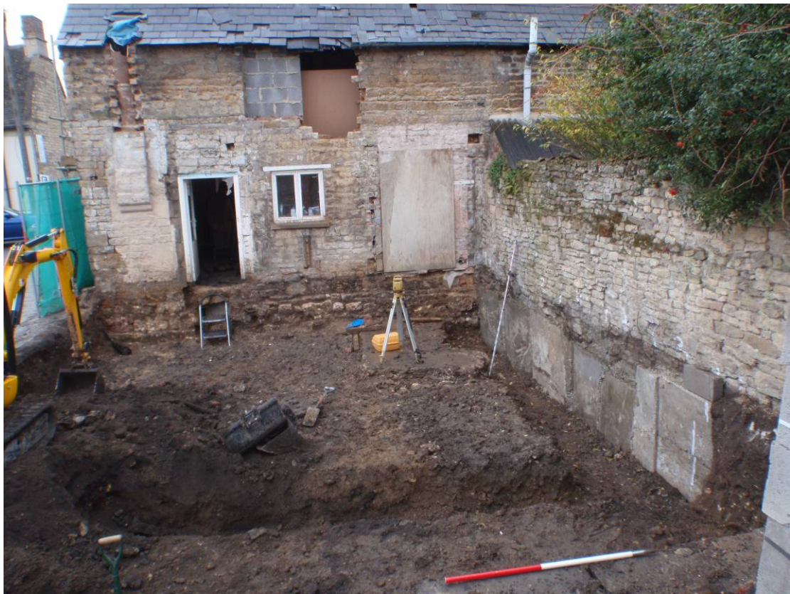
Plate 2. General view of footings looking south
