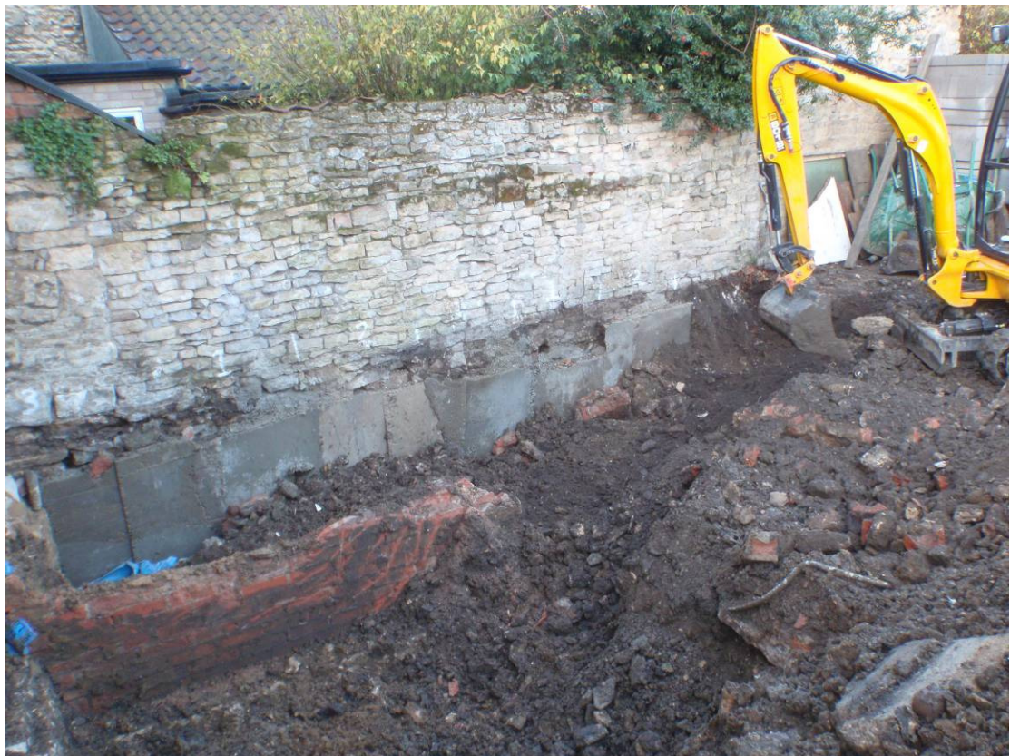
Plate 6. Excavating rubble from area of former extension, looking west
