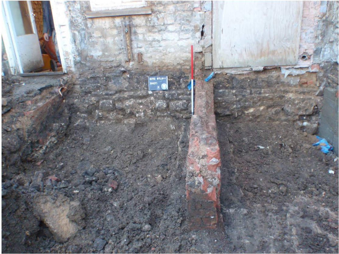
Plate 5. View showing exposed stone footings of house, and wall [002], looking south
