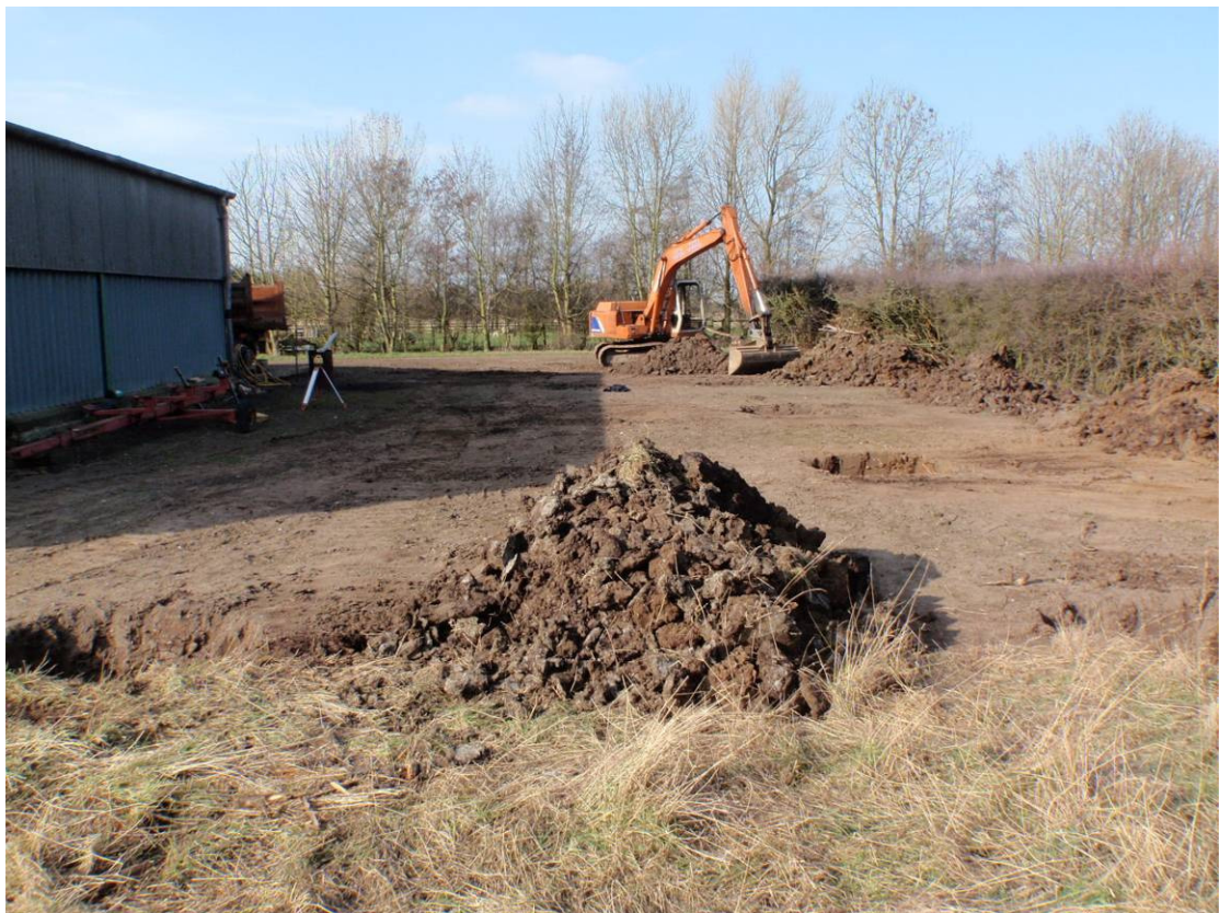
Plate 4. General view looking northwest following completion of stanchion pits
