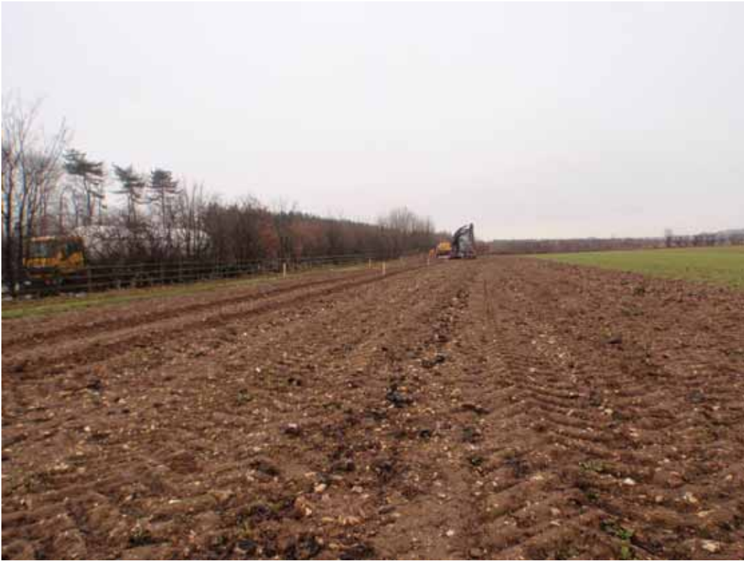
Plate 1: General view of site prior to excavation
