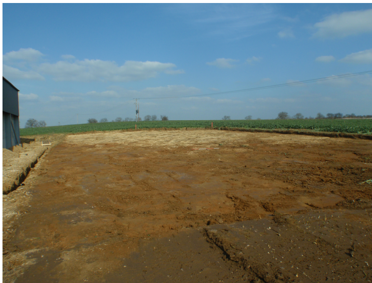
Plate 2 – The site after stripping, looking northeast
