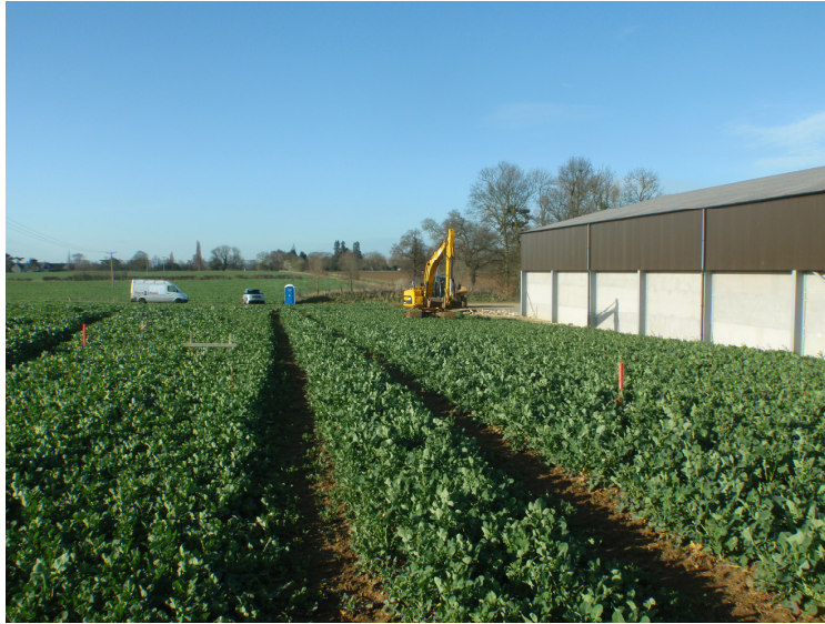
Plate 1 – General view of the site prior to works, looking southwest
