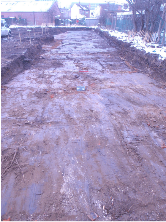
Plate 4 – Area 1 after stripping, looking west
