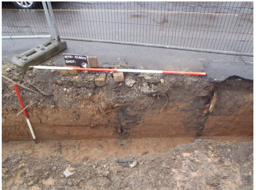
Plate 2 Section 1, features [003] & [009], looking northwest
