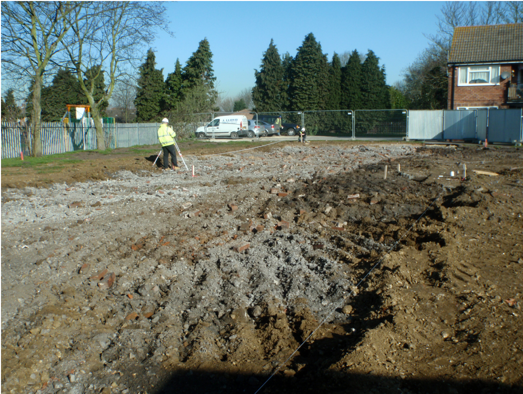
Plate 1: Location of bungalows showing demolition rubble (002/022)
