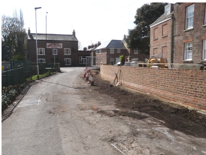
Plate 6 – View showing the road widening works, looking south
