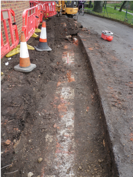
Plate 8 – Brick (012) edging of former path, looking north
