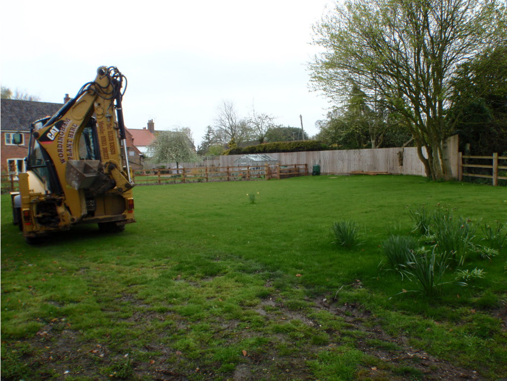
Plate 1 General view of the site from southwest corner, looking northeast
