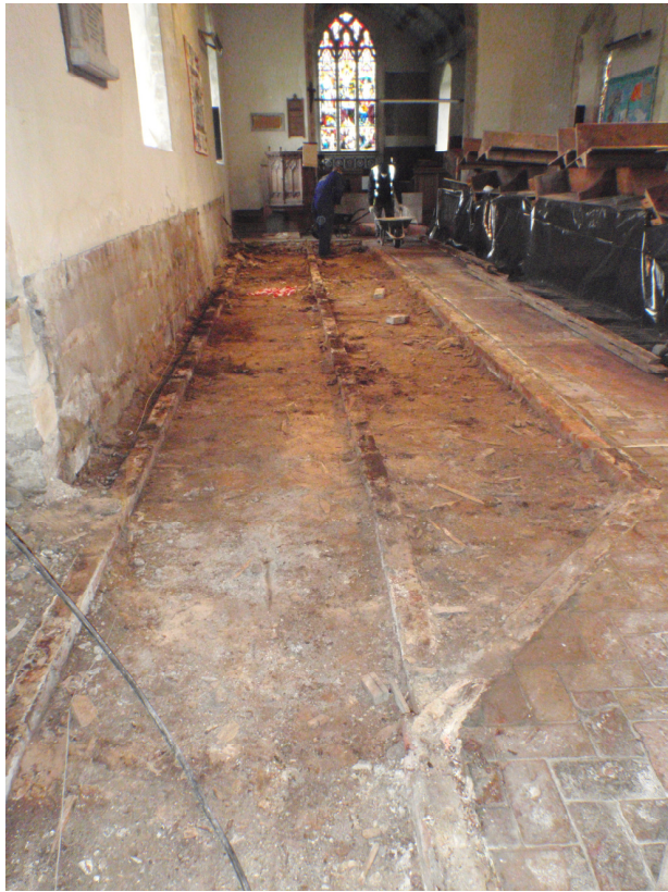
Plate 1 – View showing the area of works, looking east
