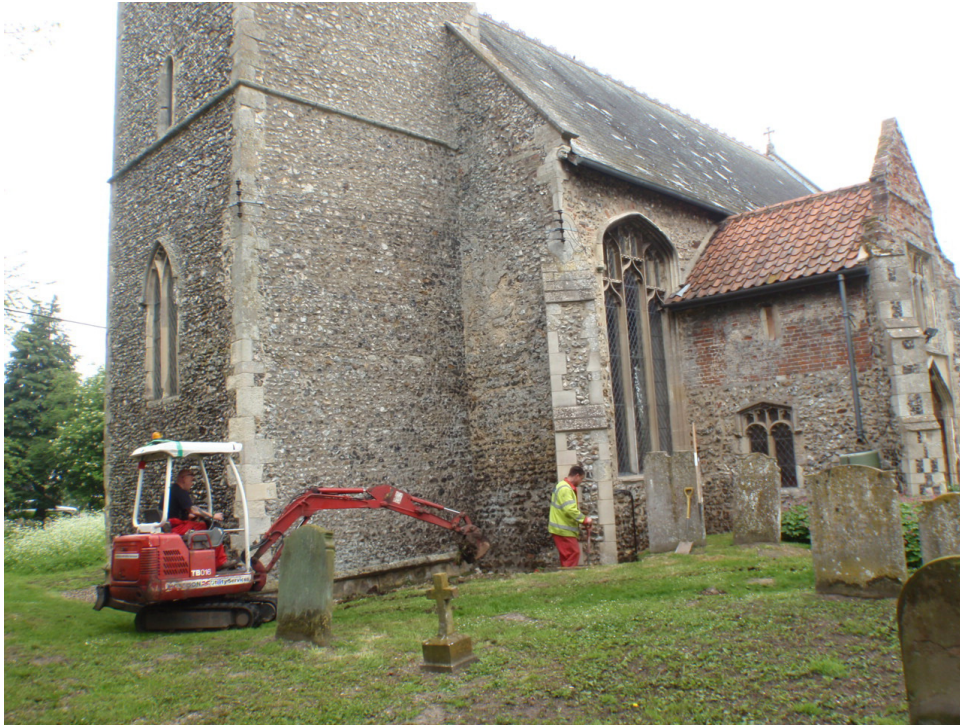
Plate 1 – General view showing the works in progress, looking northeast
