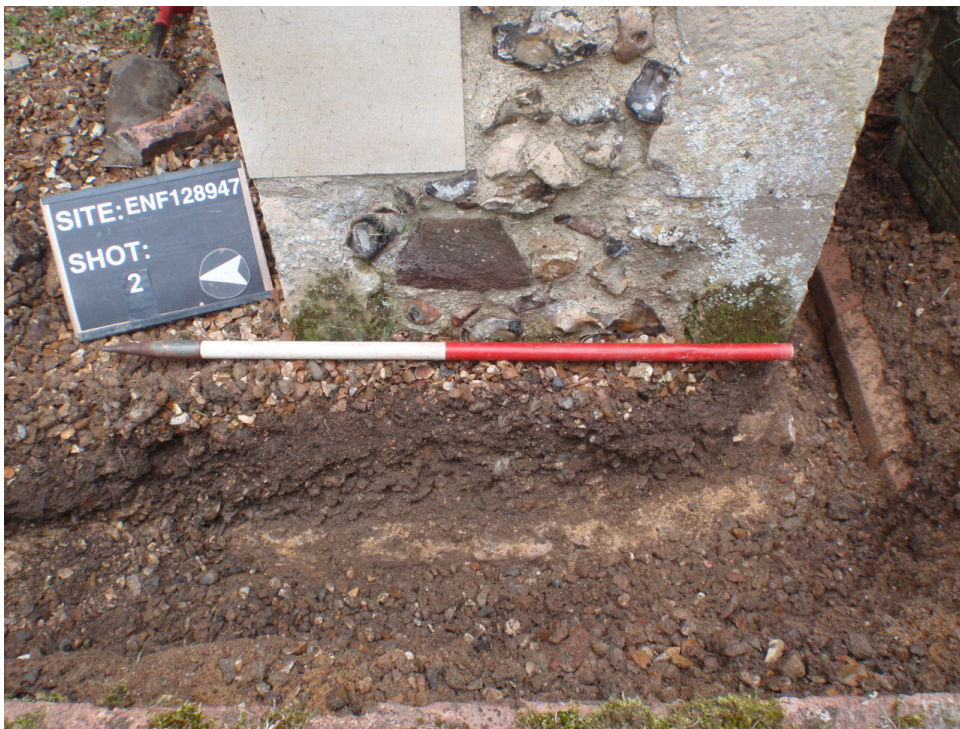
Plate 2 – Section 1 showing the exposed buttress foundation, looking northeast
